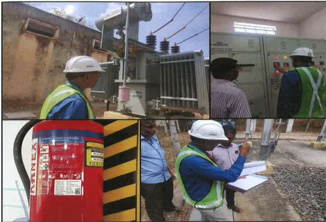
Energy conservation and Fire Safety facilities observed in the Campus
