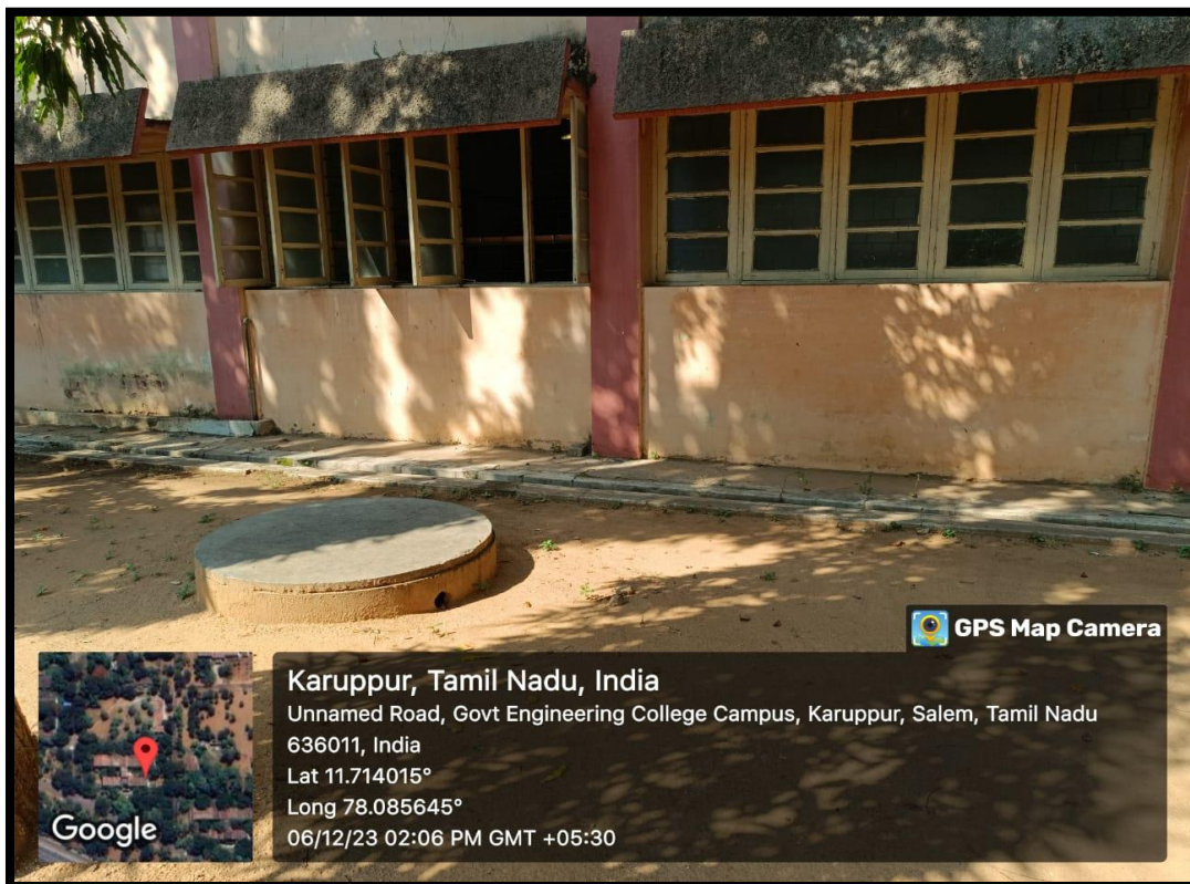
Figure 5: Rainwater harvesting Pit in Department of Metallurgical Engineering
