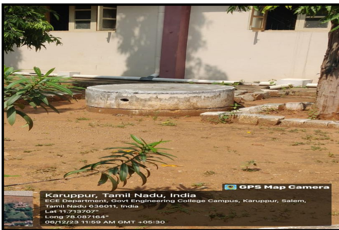
Figure 1: Rainwater harvesting Pit in Department of ECE
