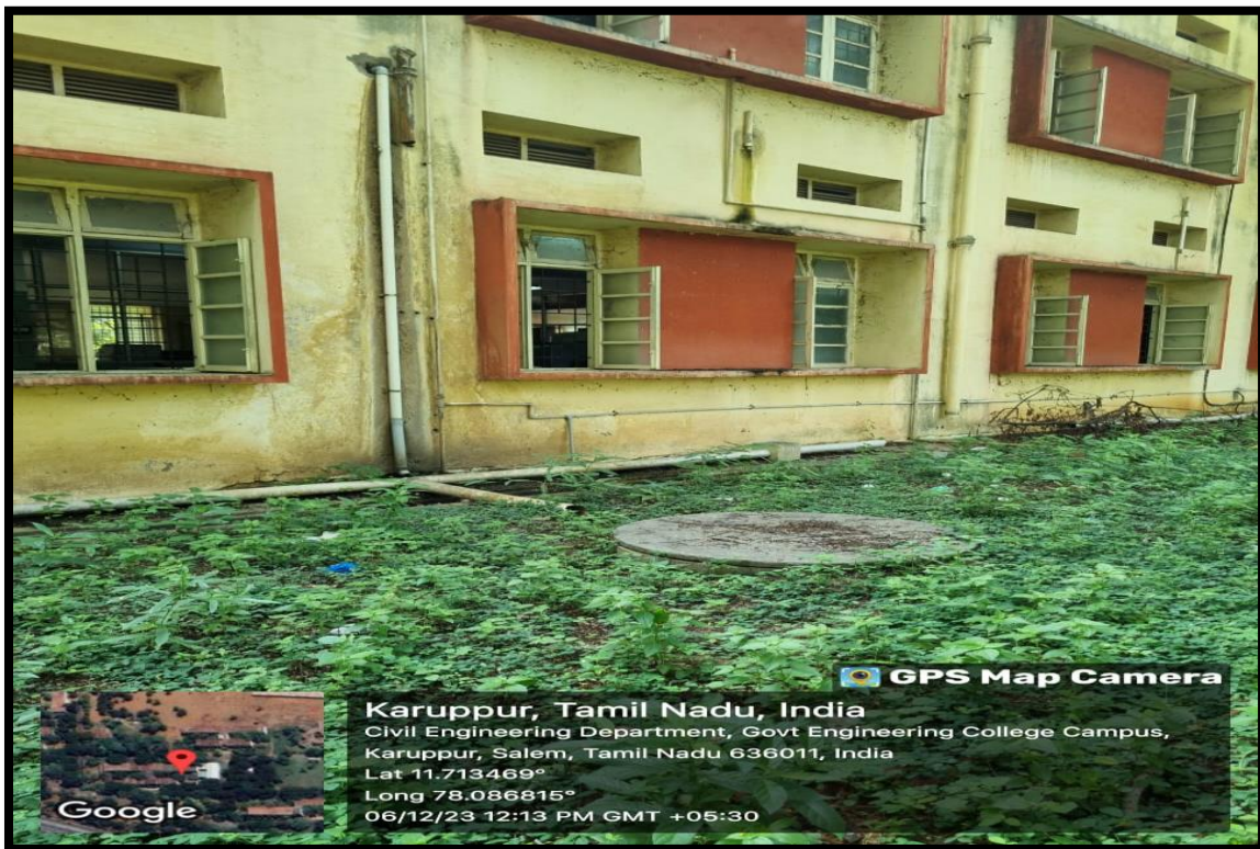
Figure 3: Rainwater harvesting Pit in Department of Civil Engineering
